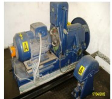
*Note the lousy wiring and encoder (tacho) for the closed-loop safety circuit conversion from 2-speed to V3F*
