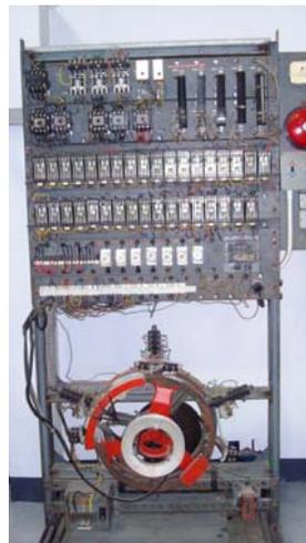
Training Facilitator Roger Marshall has to cope with the training requirements, ranging from the newly qualified lift artisans on the old relay logic equipment with rope controlled mechanical selectors (left), progressing to the latest state of the art microprocessor logic with electronic shaft information (below) for the older mechanics of yesteryear.
